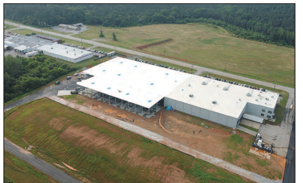
LINDE + WIEMANN U.S., Inc. – 1720 Knox Bridge Crossing Road, Lavonia, Georgia, 30553 –expansion
